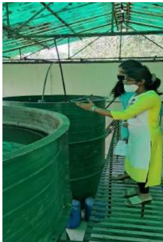
Figure 2.9 Green audit team inspecting the clarifier of ETP
