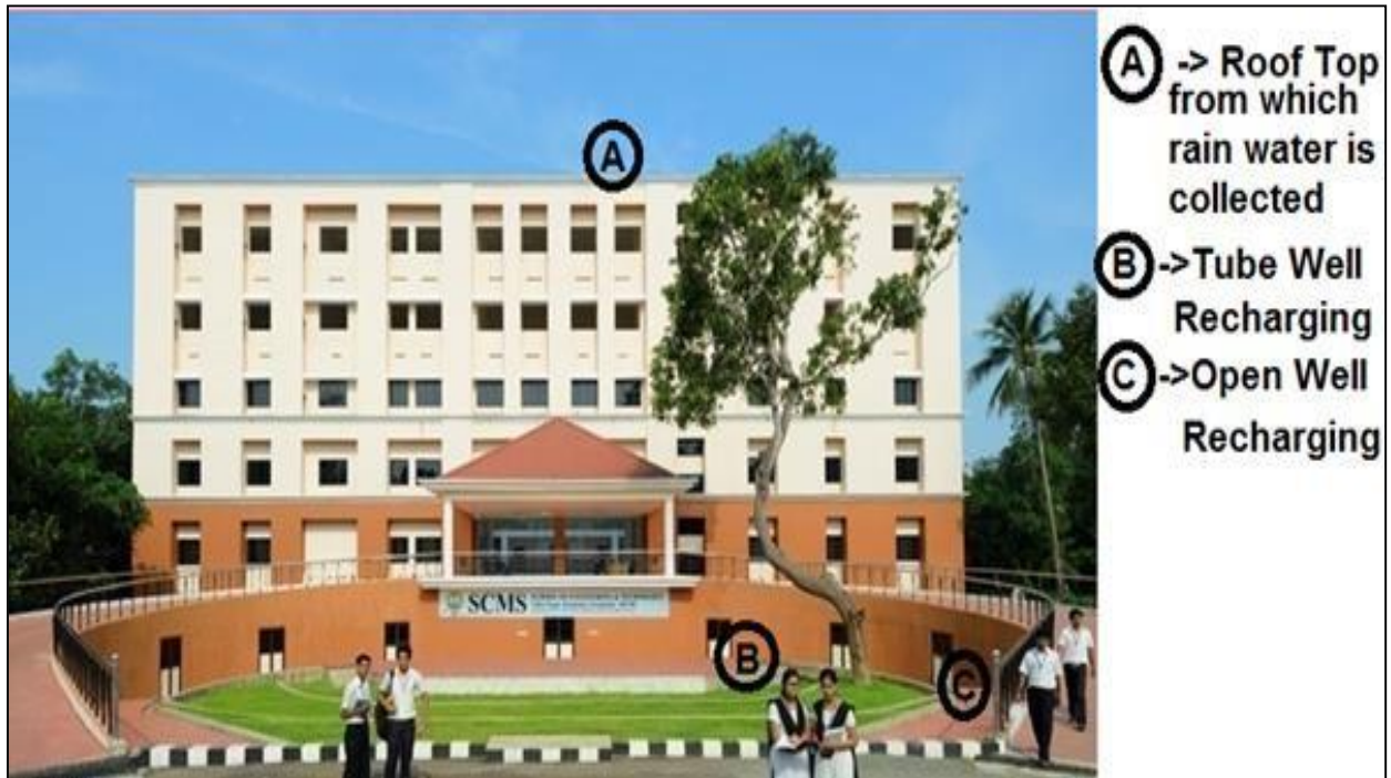
Figure 2.7 Salient locations of well recharging system at SSET
