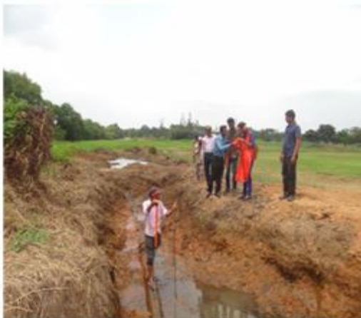
Pipeline Investigation project under German company named SEWERIN on May 29, 2019
