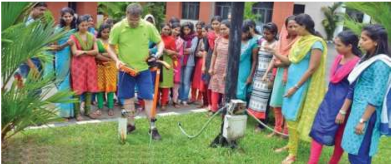
Mr. Lutz Höernschemeyer, Manager, Sewerin from Germany giving a demonstration for students of SSET to locate water pipe on October 18, 2015
