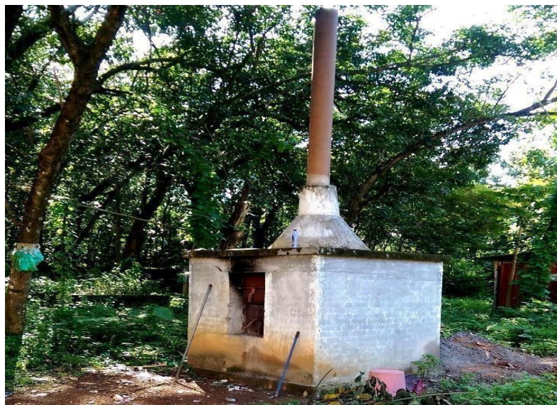
Figure 1.7 Garbage burner at SSET, Karukutty
