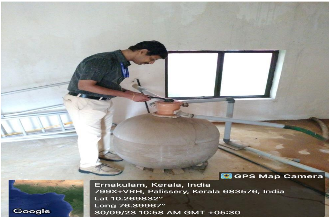
Fig. 2 Borewell recharge installation. Rain water collected at rooftop is treated using Pressure sand filter before taken for bore well recharge
