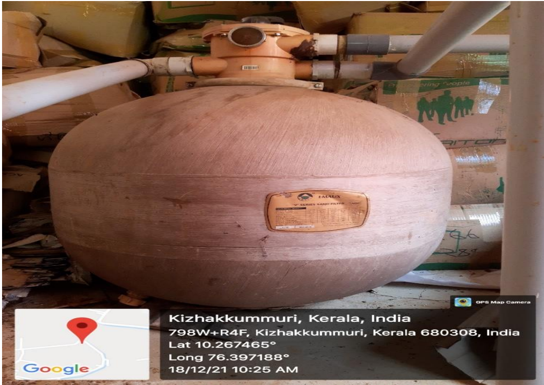
Fig. 2 Borewell recharge installation. Rain water collected at rooftop is treated using Pressure sand filter before taken for bore well recharge
