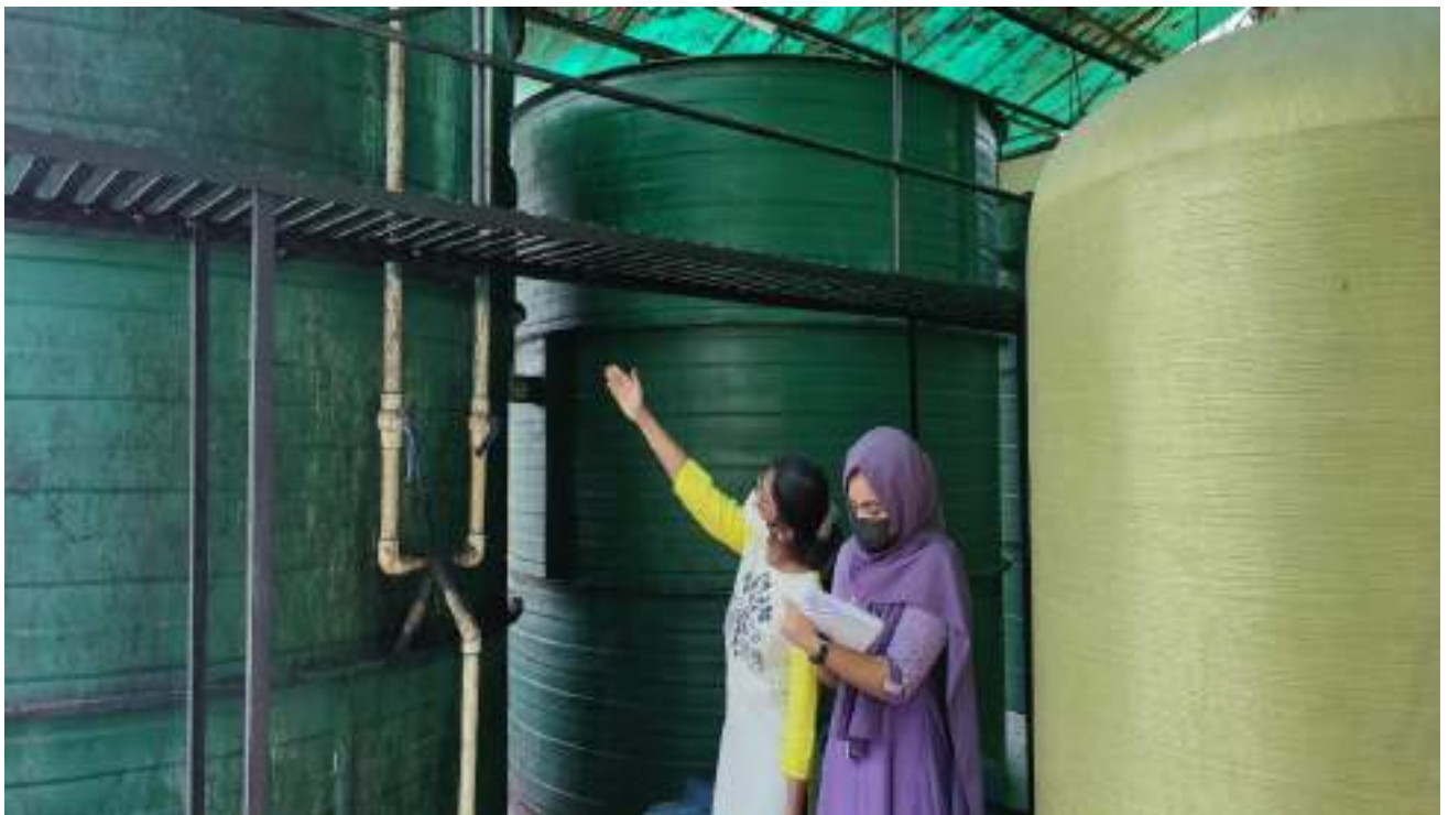
Figure 2.7 Green audit team inspecting the ETP of SSET campus
