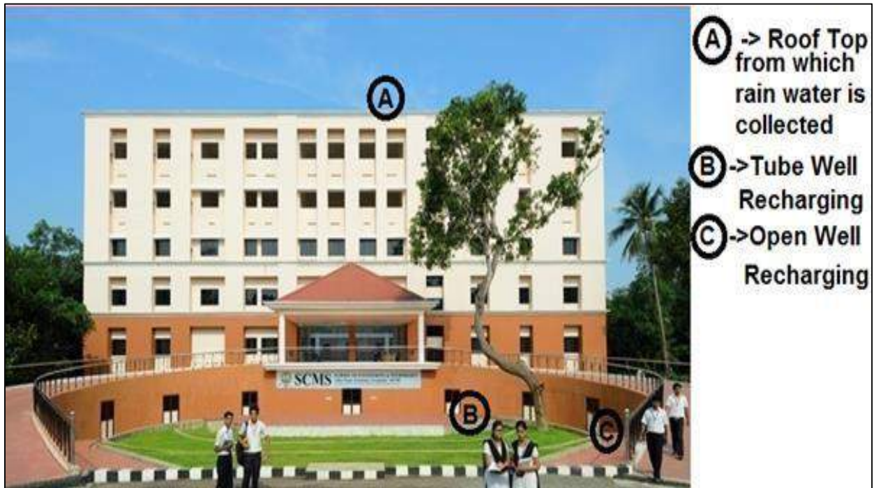
Figure 2.10 Salient locations of well recharging system at SSET
