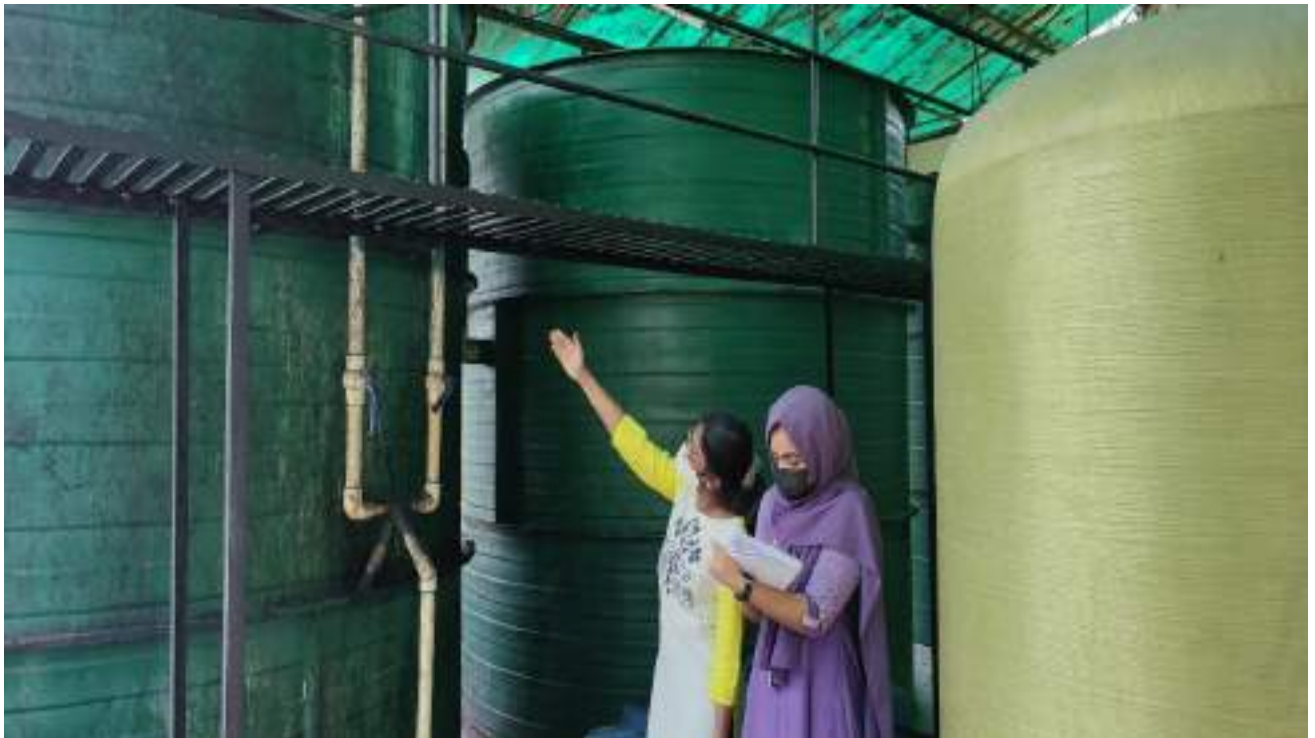
Figure 2.7 Green audit team inspecting the ETP of SSET campus
