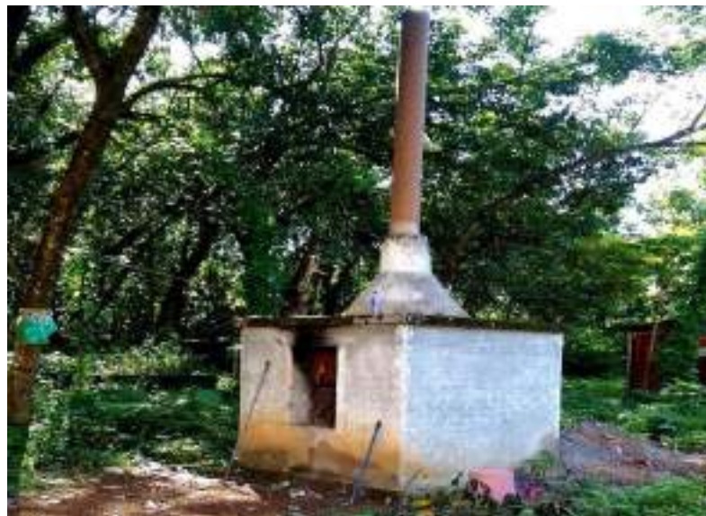
Figure 4.4 Garbage burner at SSET, Karukutty
