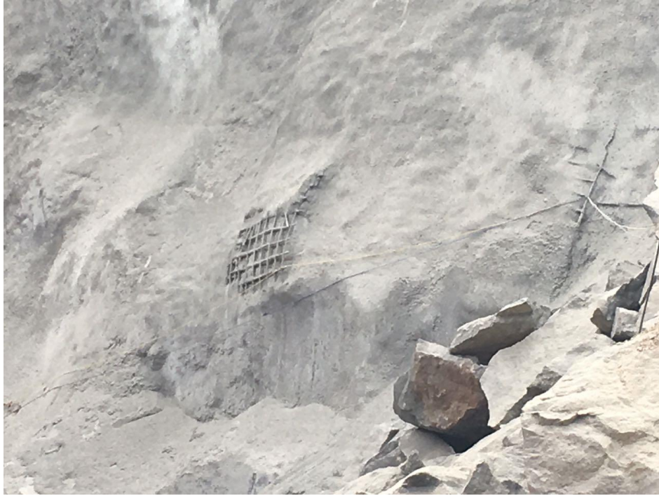
Shotcrete at periphery of tunnel
