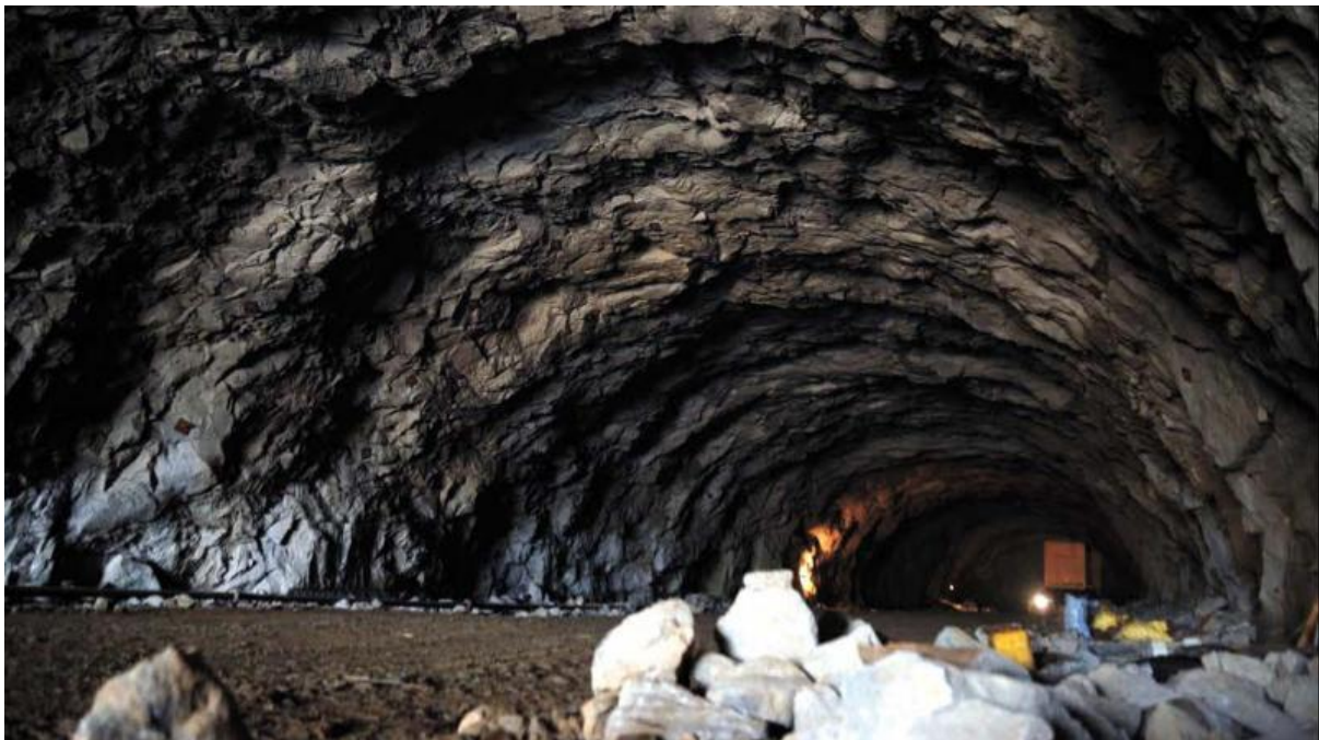
Inside view of tunnel
