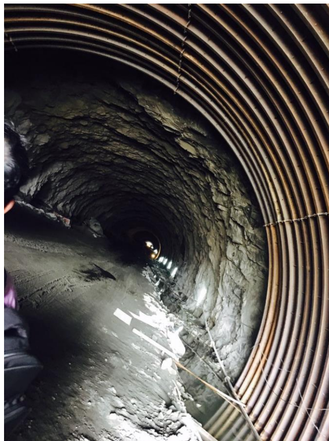
Supporting Steel frames
