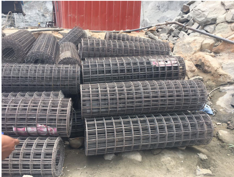
Reinforcement mesh for shotcreting
