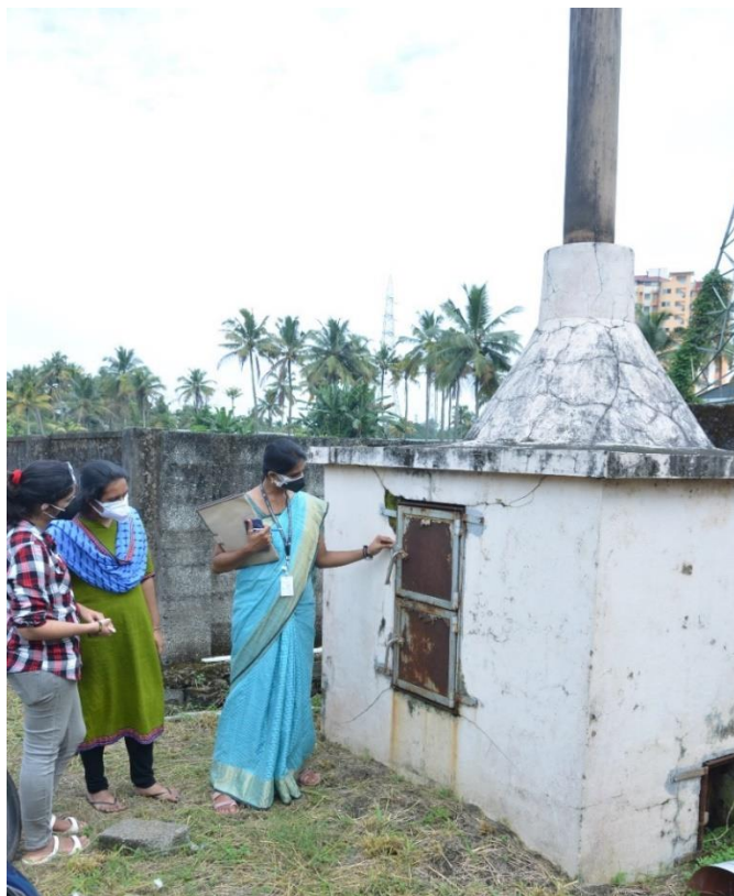
Figure 4.6 Green audit team inspecting garbage burner
