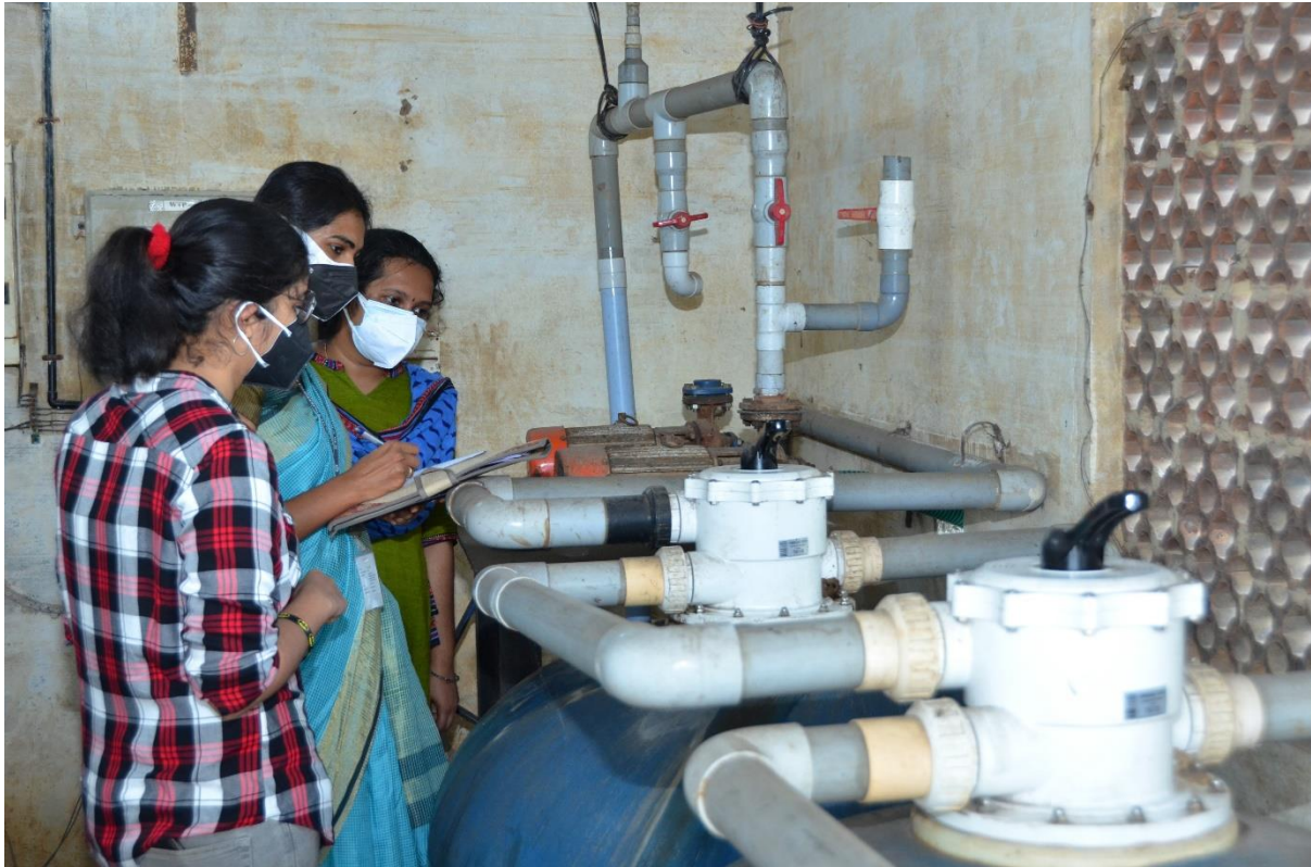
Fig.2.2 The audit team examining water treatment plant
